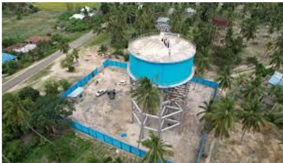
Modern water tank in Pemba.
