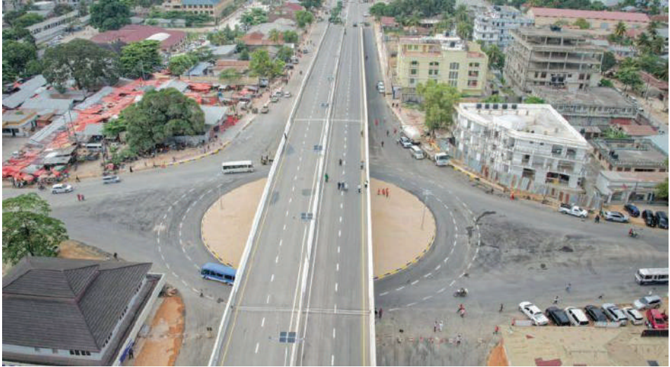
Figure 22: A 23.7 Bil. TZS Hussein Ali Hassan Mwinyi Flyover No 1 at Mwanakwerekwe
